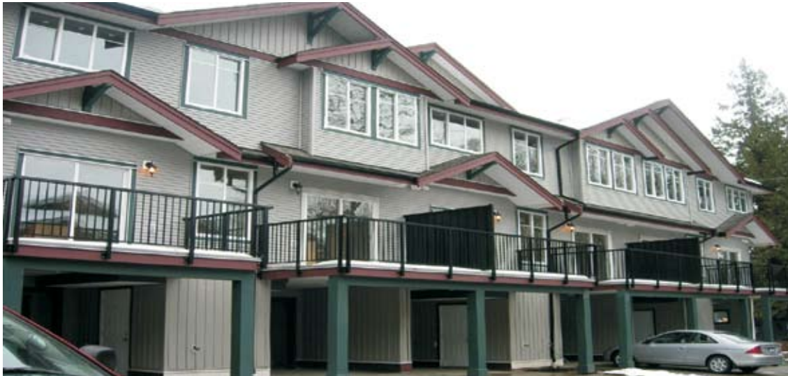
Using electric tank this townhouse project is heated with a JH 30
